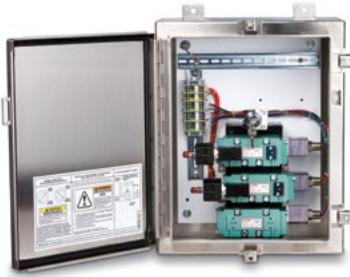
Figure 11.8 Redundant SOV
