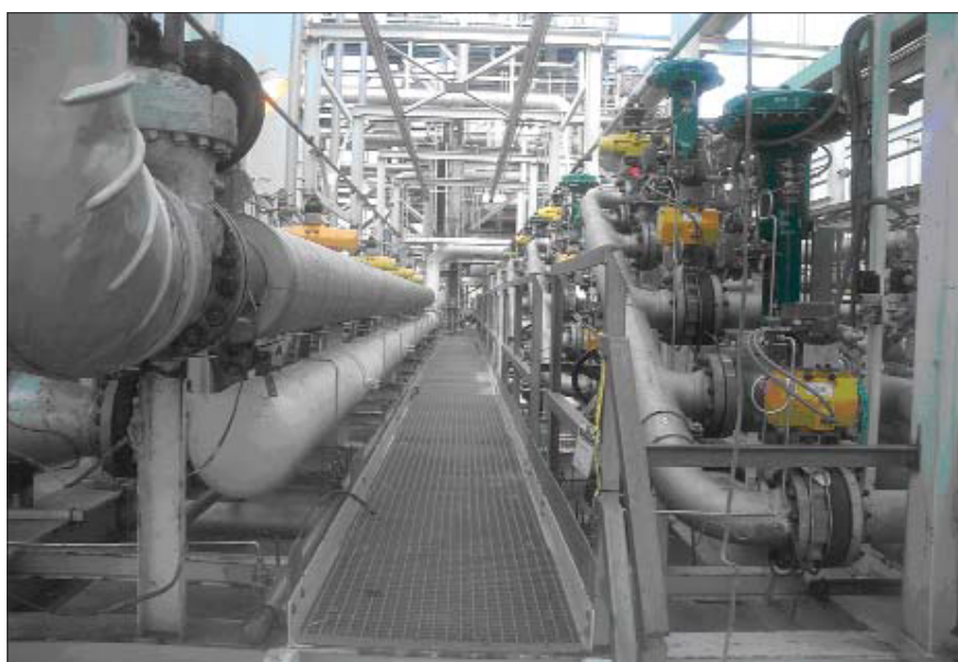
Figure 4 This PSA skid was producing only 65-70% hydrogen. Replacing the valves improved production by 20%
