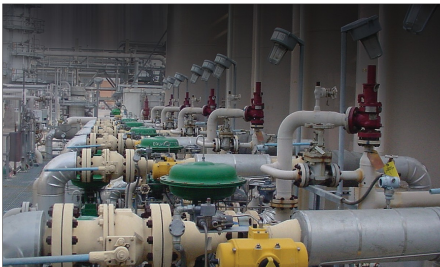
Figure 1 PSA control valves have stringent requirements for stroking frequency and shut-off
