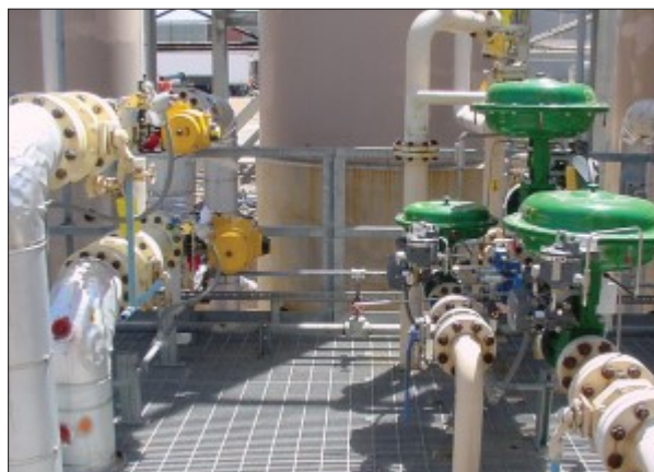
Figure 3 To cure PSA problems at an Oklahoma refinery, Fisher GX globe valves and high performance butterfly valves were installed
