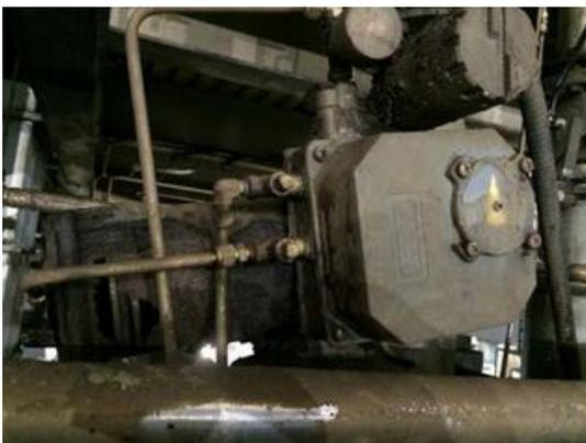
*(TOP VIEW) The existing actuator experienced significant damage due to the harsh operating environment.*
