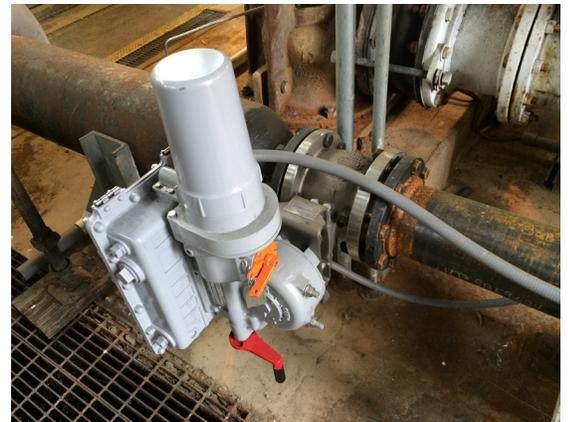
(TOP VIEW) Fisher V150 control valve with EIM M2CP electric actuator
