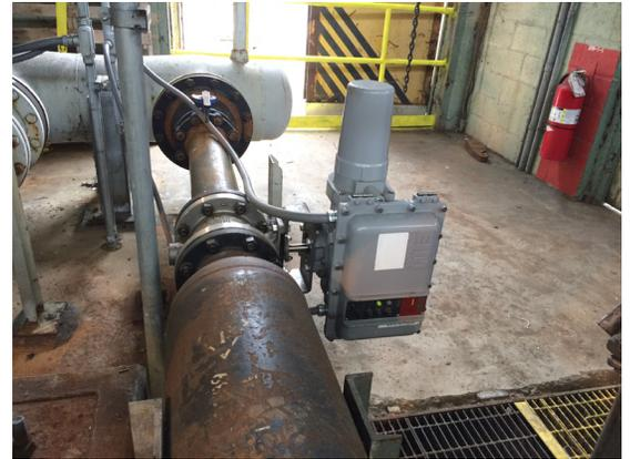
(SIDE VIEW) Fisher V150 control valve with EIM M2CP electric actuator
