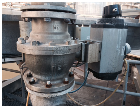
The upstream seat provided improved (Class VI) shutoff, while the downstream seat provided a scraping/wiping action of the ball
